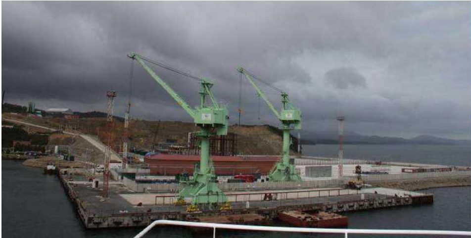
Figure 3 Reactor Compartment Long-term Storage Facility
