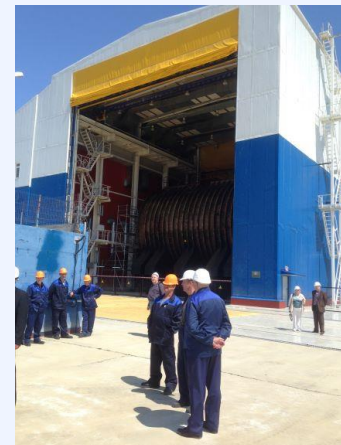
Blast and Paint Facility
