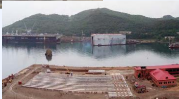
Onshore storage facility at Saida Bay started into operation in 2006 (top left) and that at Razboynik Bay at around the same time (bottom right) .
